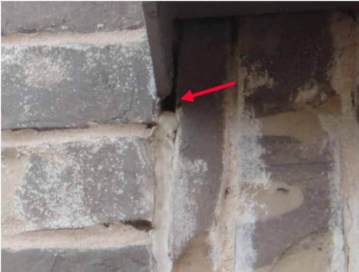
North brick expansion joint has incomplete sealant at top resulting in small opening - minor repair (See photo)
