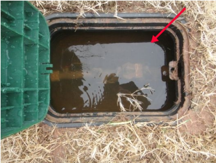
Note: Sprinkler system backflow preventer valve located in front yard valve box ( See photo ) - valve box full of standing water at time of inspection - discuss
