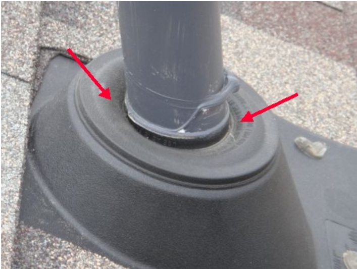
1 north plumbing vent roof jack has rubber seal inverted - will hold water - not typical - minor repair (See next photo)
