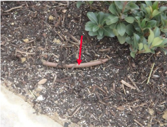
Exposed drip line in flower bed south of driveway - subject to damage - condition minor (See photo)
