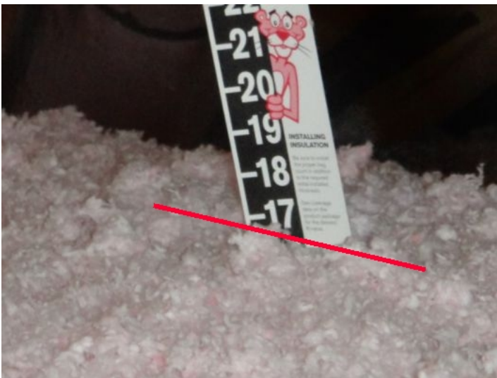
Note: View of insulation installers depth marker
