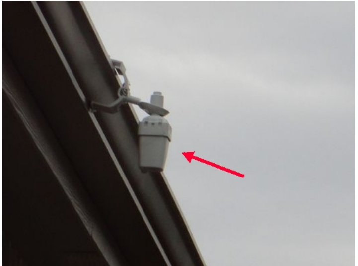
Note: Sprinkler system Rain Sensor located at south roof edge (See photo)
