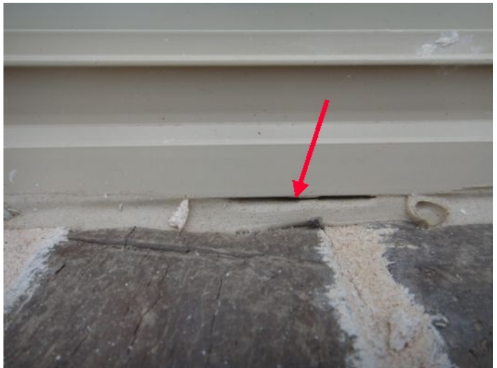
Window frame to brick caulking failed / incomplete at random - minor repair (See photos)
