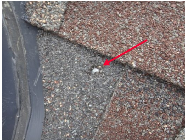
Unsealed roof fasteners near east chimney vent flashing - minor repair (See photo)
