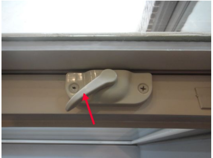
Some windows require excessive force to close latches when in full down position - not typical (See photo) - 2 of 3 windows in den, 2 of 4 in master bedroom, study LH window
