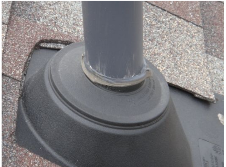
View of properly installed roof jack seal
