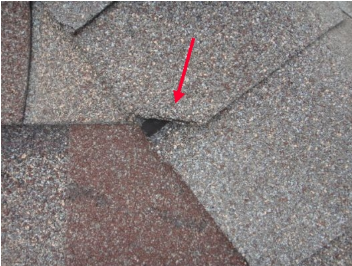
1 damaged shingle at NE ridge line - condition minor (See photo)
