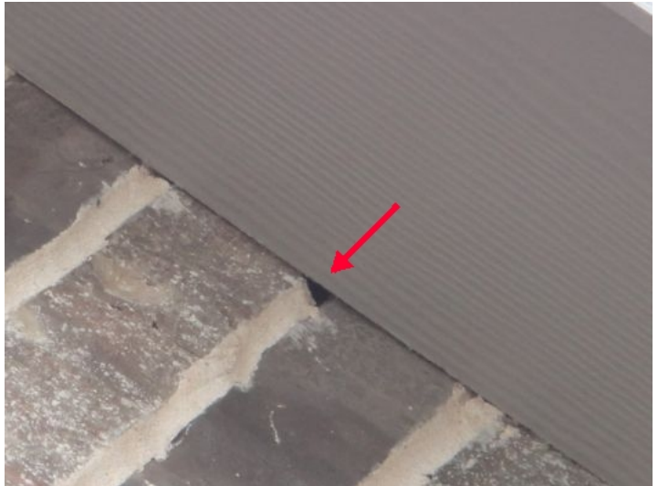
Small areas of missing / incomplete brick mortar resulting in small openings where soldier bricks meet frieze board trim - minor repair (See photos)
