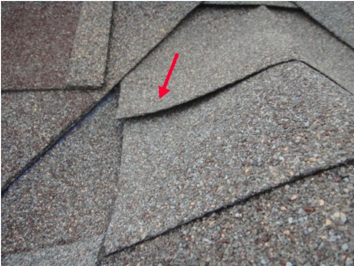
Several areas of uplifting ridge shingles are prone to wind damage (See photos)
