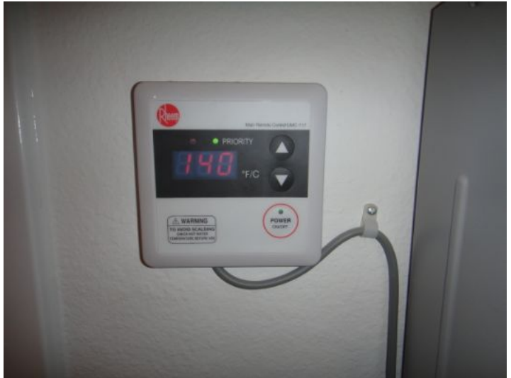
Note: Water heater temperature control panel located at garage wall (See photo)
