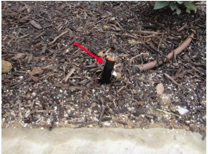
Zone 3 has 1 head that extends but does not spray at flower bed south of driveway (See photo)
