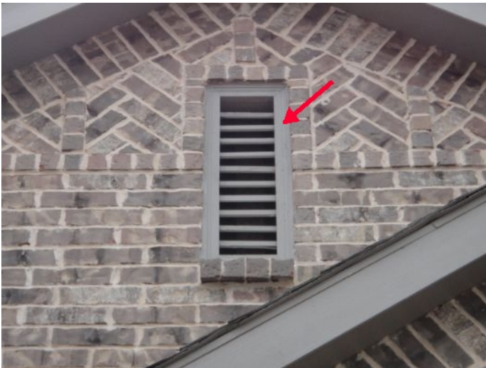
Note: Decorative wood gable vents will require regular maintenance to prevent water damage - discuss (See photo)
