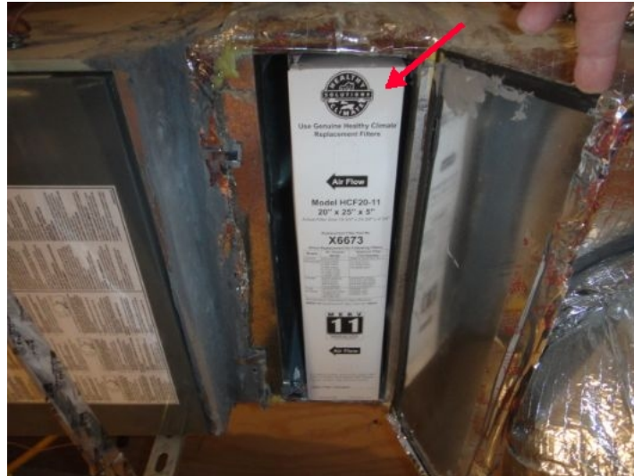
Note: Air filter changed at air handler unit in attic (See photo)
