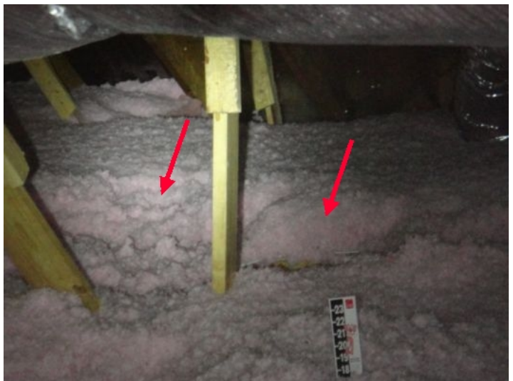
Blown ceiling insulation is loose / disturbed at areas above den caused by worker foot traffic - no longer at posted depth in this area - discuss with client (See photo)
