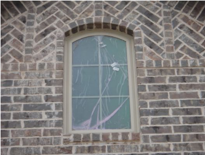
Attic window above driveway has plastic covering installed but appears cracked - consult builder (See photo)
