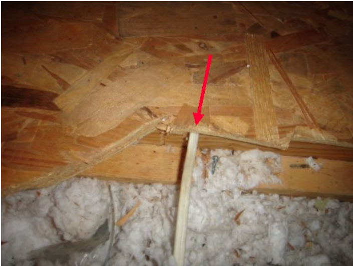
110 volt wiring pinched by added wood flooring decking in north attic - not typical - potential hazard - needs repair - discuss with client (See photos)
