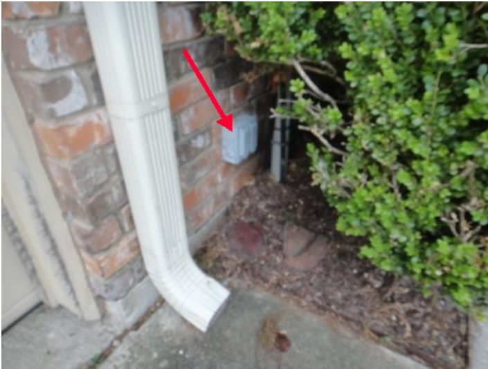
Added exterior outlets near garage are not GFCI protected as required at time of construction - potential hazard (See photo)
