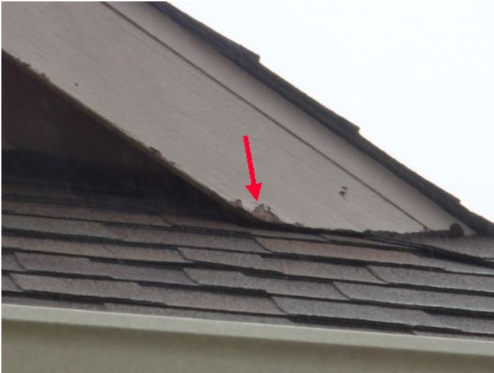
Damaged area to wood siding at west roof gable above front patio - possibly caused by hail strikes - discuss (See photos)
