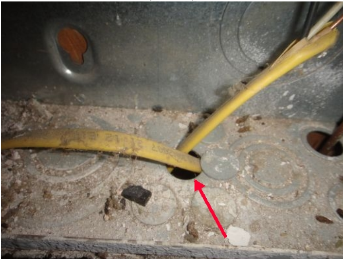
Added wiring exits electric panel with no feed through fittings installed - purpose of feed through fitting is to prevent abrasion to wiring - minor repair ( See photo )
