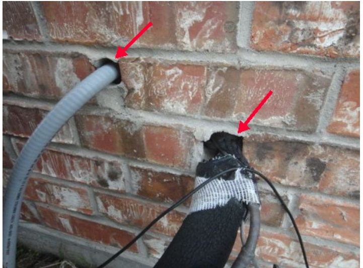
Air conditioner electrical and refrigerant lines are not sealed at brick penetration (See photo)
