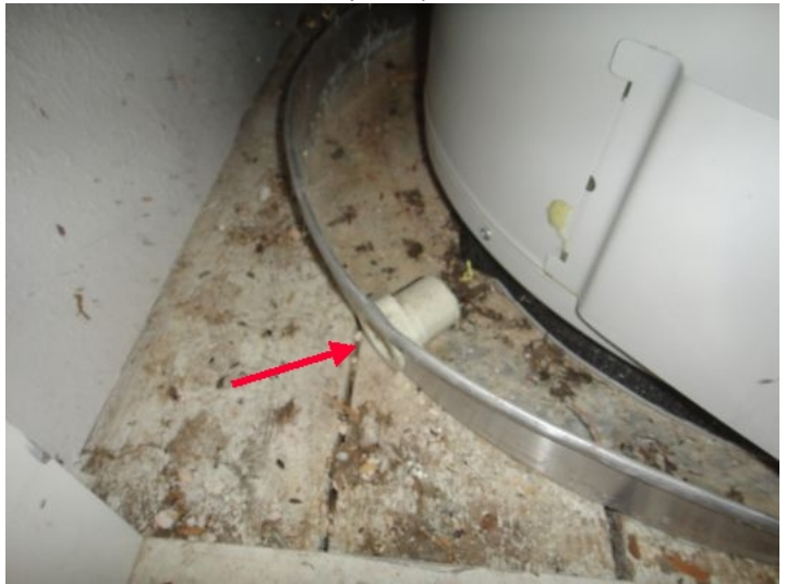
Garage water heater overflow pan does not have drain line to exterior ( See photo ) - discuss code change
