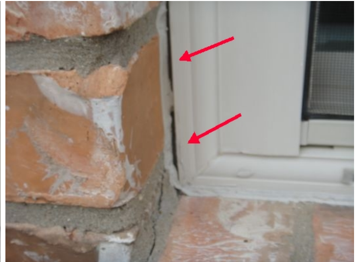
Minor separation of brick at south window opening
