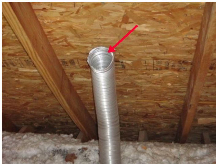
Bathroom exhaust fans vent directly into attic space as allowed at time of construction - current code requires vents to terminate at exterior of structure.
