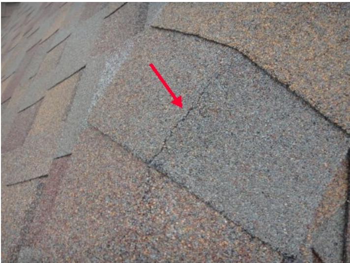
Random areas of split / cracked ridge shingles - recommend to seal (See photos)
