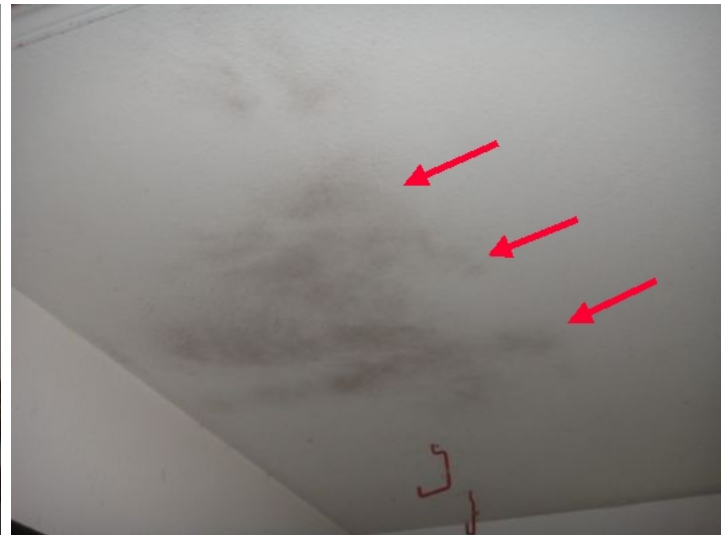
Note: Discoloration at garage ceiling area - cause not determined - consult seller (See photo)
