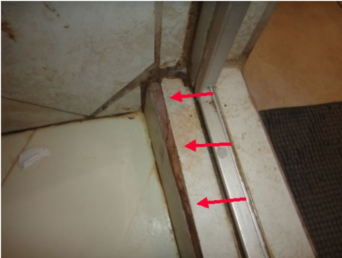
Master bath shower tile wall has failed grout / caulk at random, loose unbonded tiles at door threshold areas typical of age - discuss & show to client (See photos)
