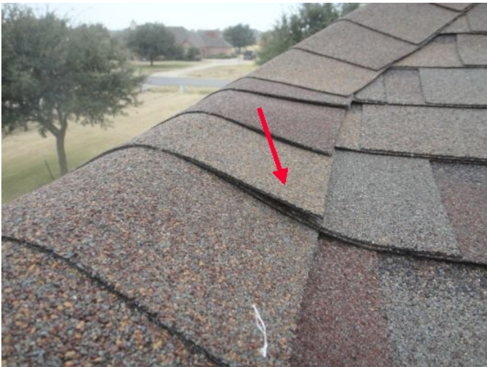
Random uplifting shingles are prone to wind damage ( See Photos )
