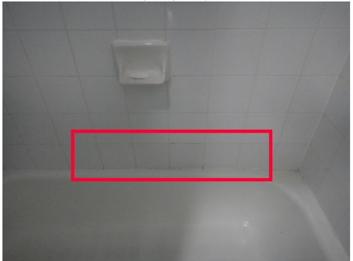
SW hall bath shower tile wall needs caulking repair at random areas & has some tiles starting to unbonded at lower rear wall area (See photo) - discuss age with client
