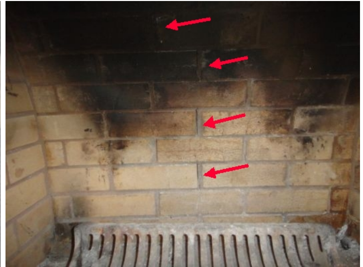
1/8 inch masonry cracks were present at rear firebox wall and is in need of corrective action (Difficult to see in photo)
