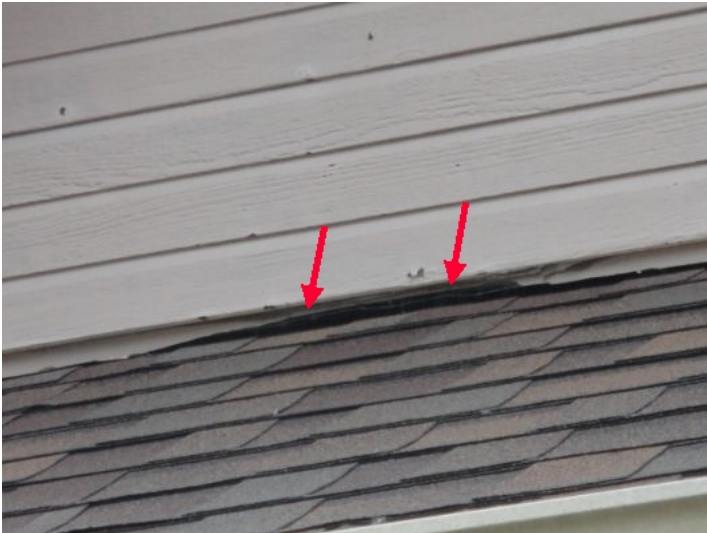
West metal counter flashing uplifting above front patio - can result in leakage - needs proper securing (See photos)
