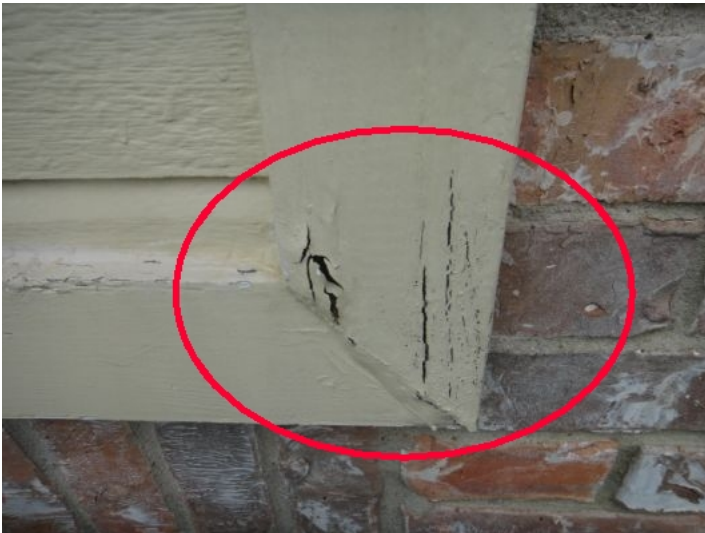
Water damage to master bath window trim (See photo)
