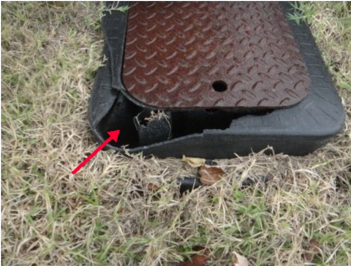
Note: Plastic water meter box in front yard shows physical damage - but functional (See photo)
