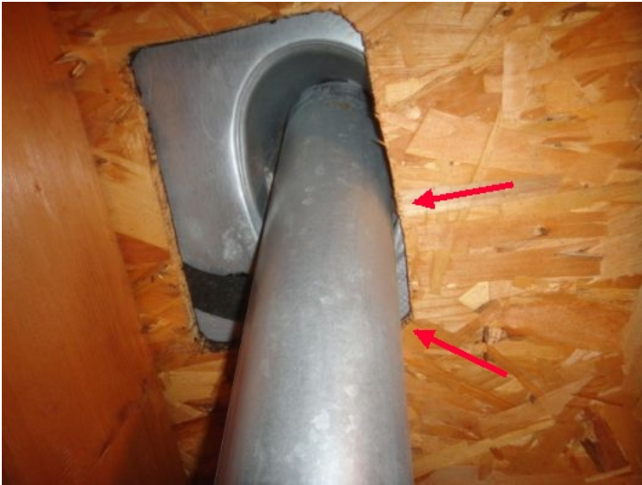
Water heater gas vent pipe in contact with wood roof decking in attic - Fire Hazard - Type "B" gas vent pipes require 1 inch clearance to combustibles - General Repair (See photo)
