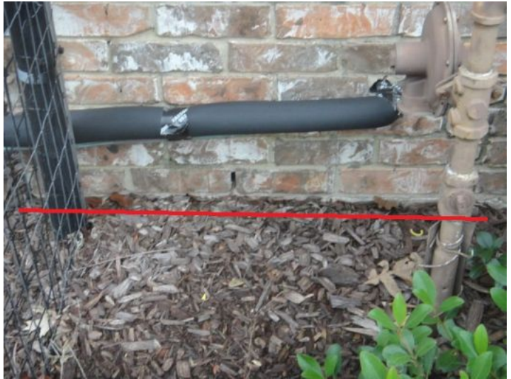
Foundation perimeter grade too high ( above brick line ) at random flower bed areas and at pool equipment area - finished grade should be maintained 2 to 4 inches below brick line - this could force water penetration during heavy rain event (See photos)
