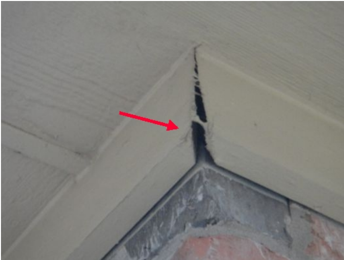
3/8 inch separation of frieze board trim at SW corner
