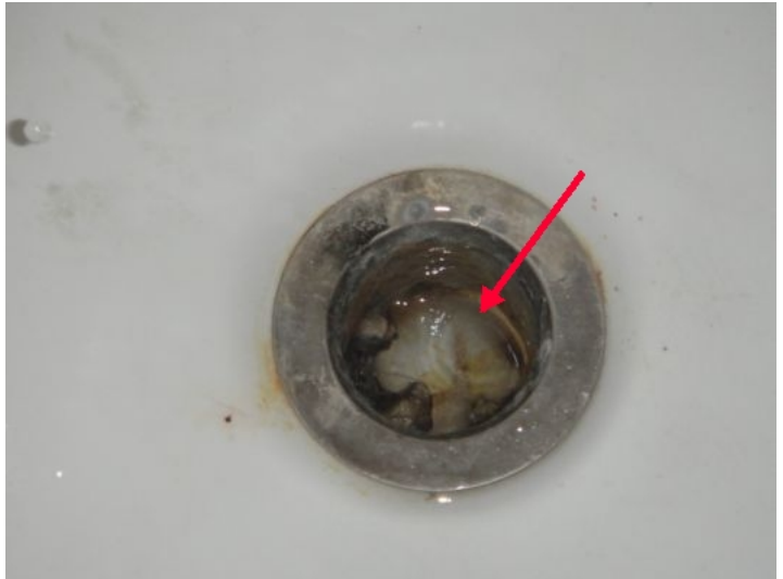
SW hall bath tub drain fitting shows obvious corrosion with missing sections - cannot connect drain stop as intended (See photo)
