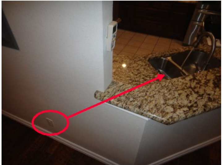
1 living room wall outlet is within 6 feet of kitchen sink & is not GFCI protected (See photo)
