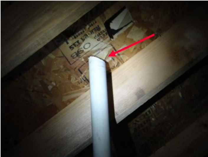
Observed 1 plumbing vent stack in north attic area does not penetrate roof as intended - this can result in sewer gas entering attic space (See photo)
