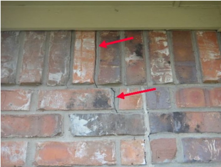
Brick mortar crack at south expansion joint area
