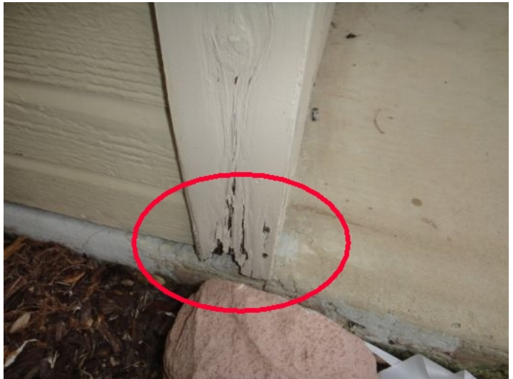
Water damage to vertical wood trim at end of front patio (See photo)
