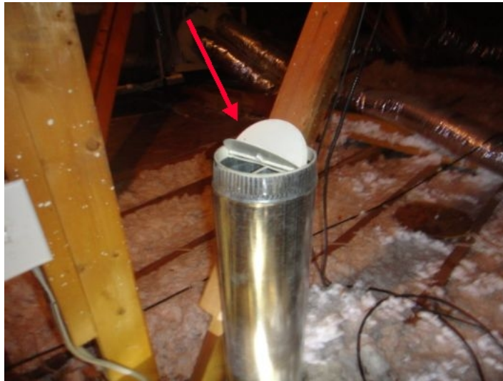
Range vent was terminated in the attic - not typical - should vent to exterior (See photo)
