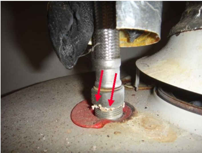
Garage water heater shows evidence of seepage at hot water line connection point (See photo)
