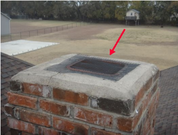
Chimney top does not have a rain cap or spark arrestor installed - not required at time of construction but recommended ( See photo )
