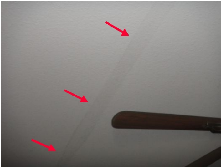
Note: Minor water stain across study ceiling - no evidence of current leakage noted - consult seller for leak / repair history (See photo)
