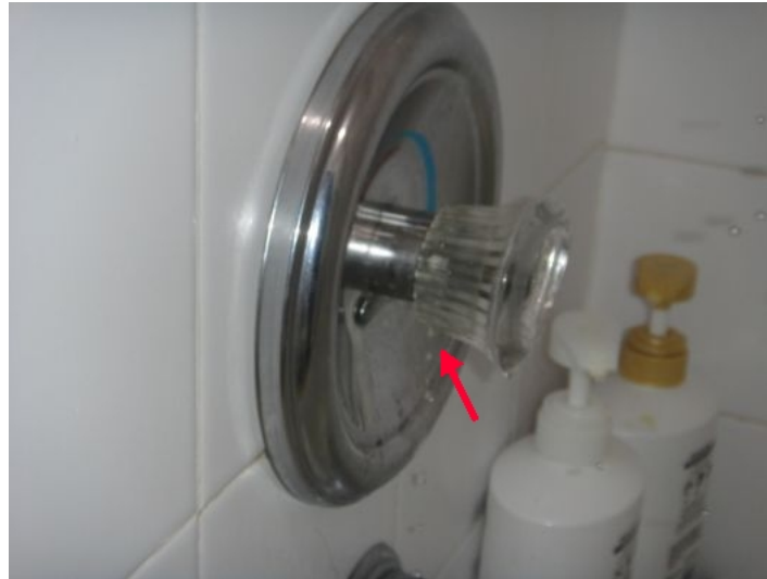
SW hall bath shower mix valve leaks at control stem from behind plastic knob when on - not typical (See photo)
