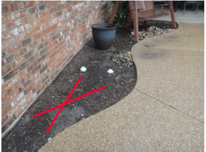
Low areas with evidence of water ponding at rear flower bed areas (See photos)
