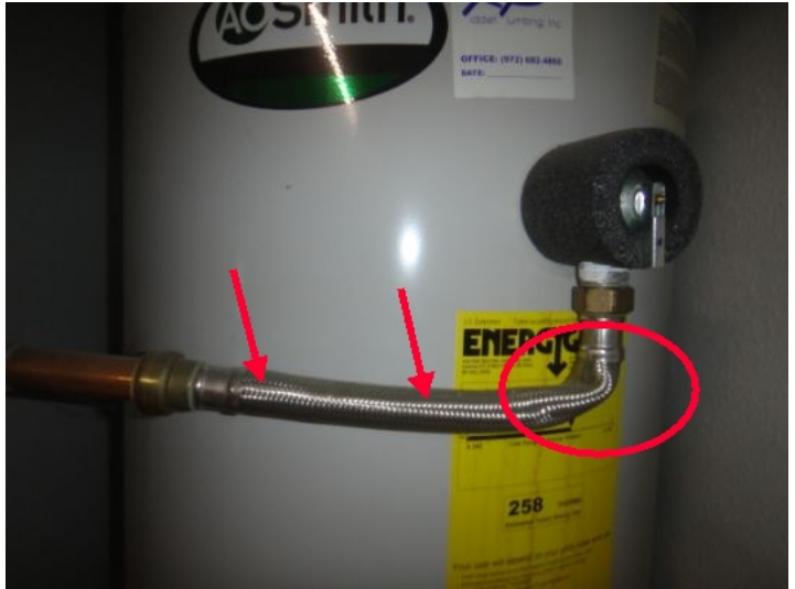
Garage water heater TPR valve connected with non approved flexible hose & is kinked restricting inside diameter - needs repair - Copper or CPVC pipe recommended (See photo)
