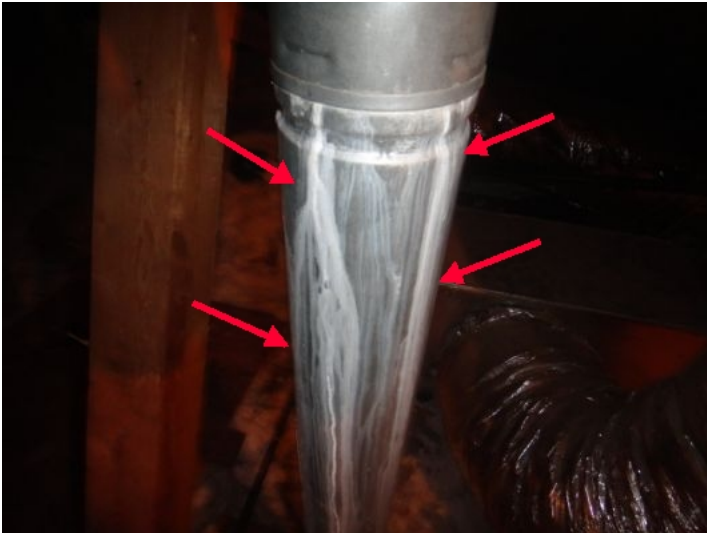
Water heater vent shows evidence of previous leakage (See photo)
