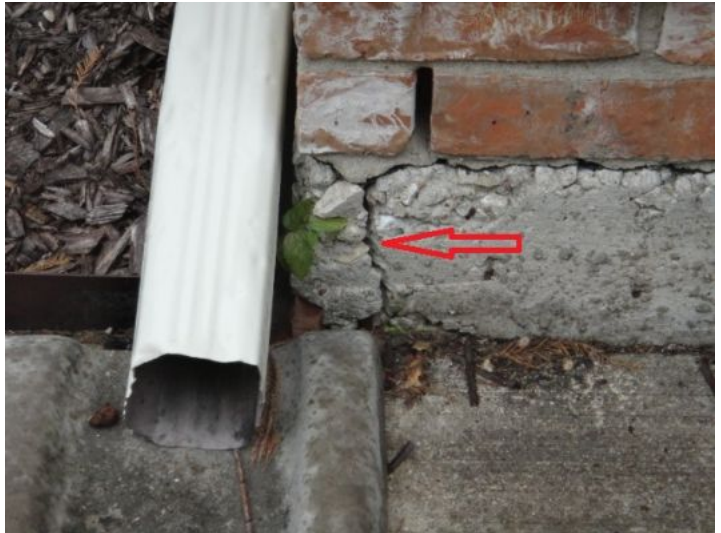
Note: Observed foundation corner breaks caused by seasonal flexing of foundation - not uncommon for age - not a structural concern ( See photo )
