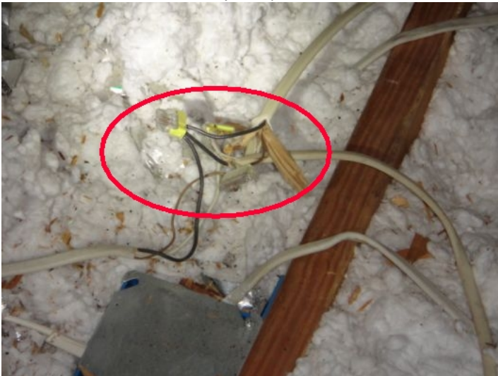
Exposed 110 volt electrical connections not in junction box in attic as required - potential hazard (See photo)
