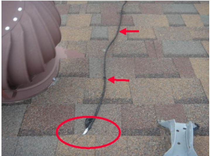
Abandoned / unused TV coax exits attic through shingle layer at east - not typical - can result in leakage (See photo)
